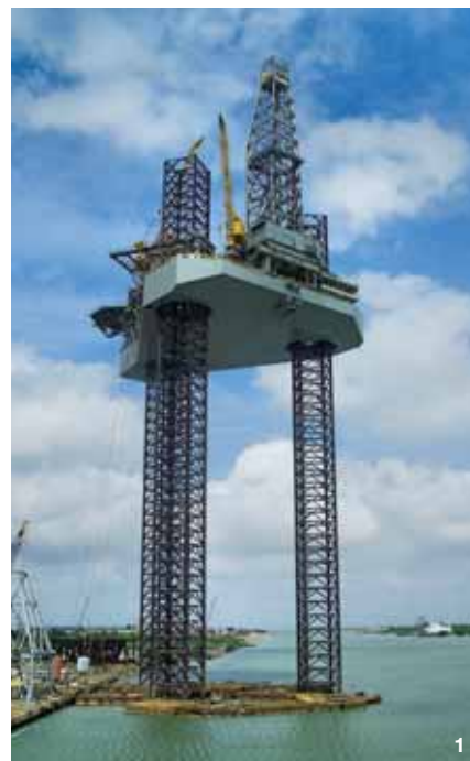
1 The Offshore Courageous is an ultra premium jackup drilling rig built by Keppel AmFELS in Brownsville, Texas for Scorpion Offshore.
