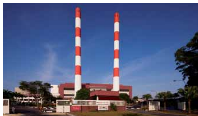
The Senoko WTE Plant can treat 2,400 tonnes of waste per day.
