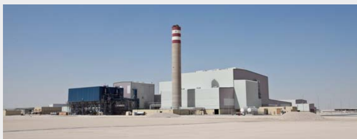
In January 2011, construction of the Qatar Domestic Solid Waste Centre project was completed and the incineration plant started burning solid waste.
