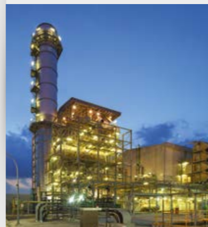
1.3 Combined-cycle gas turbine power plant
