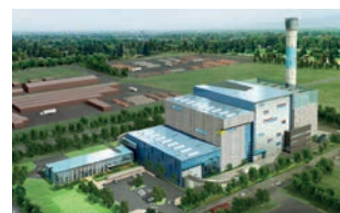
Australia's first WTE plant in Kwinana will use Keppel Seghers' proprietary technology and processes.
