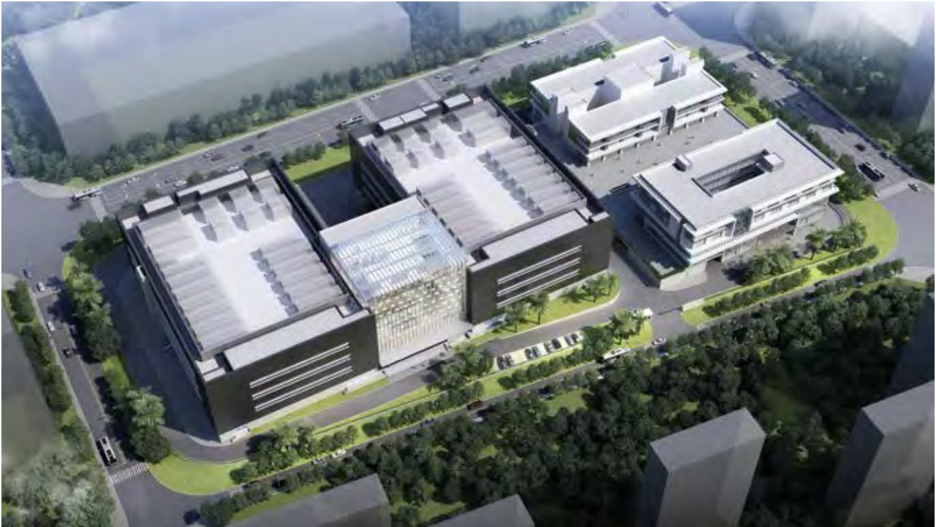
Alpha DC Fund entered into the fast-growing data centre market in China with the development of a greenfield data centre in Tonghu Smart City in Huizhou, Guangdong.
