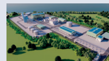
Keppel Sakra Cogen Plant Singapore's first hydrogen-ready and most advanced power plant
