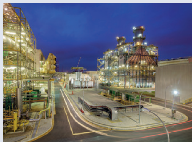
Keppel is a strong operator with a track record for engineering, developing and operating specialised assets, including Keppel Merlimau Cogen, a 1,300 MW Combined Cycle Gas Turbine power plant in Singapore.
