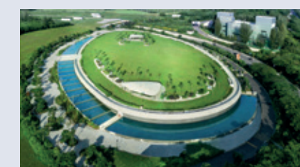
Keppel Marina East Desalination Plant Singapore's first large-scale, dual-mode desalination plant that treats both rainwater and seawater
