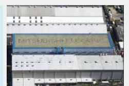
Newly built stator outer frame plant
