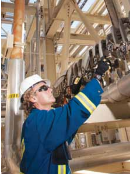
OPERATOR ADJUSTING VALVES AT THE WEYBURN FACILITY
