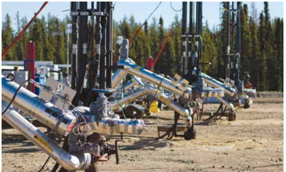
WEDGE WELLS AT FOSTER CREEK
