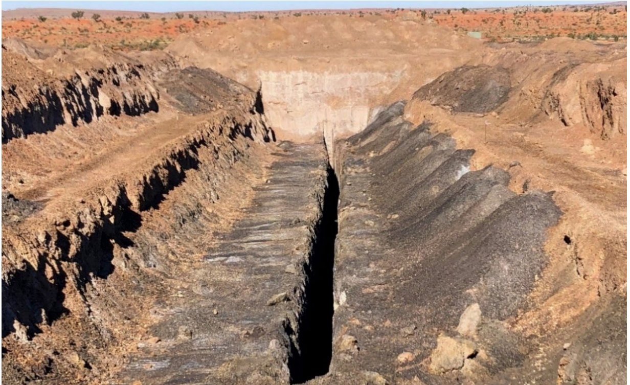
Image 5 | Trenching of the heap leach at the Nifty Copper Project
