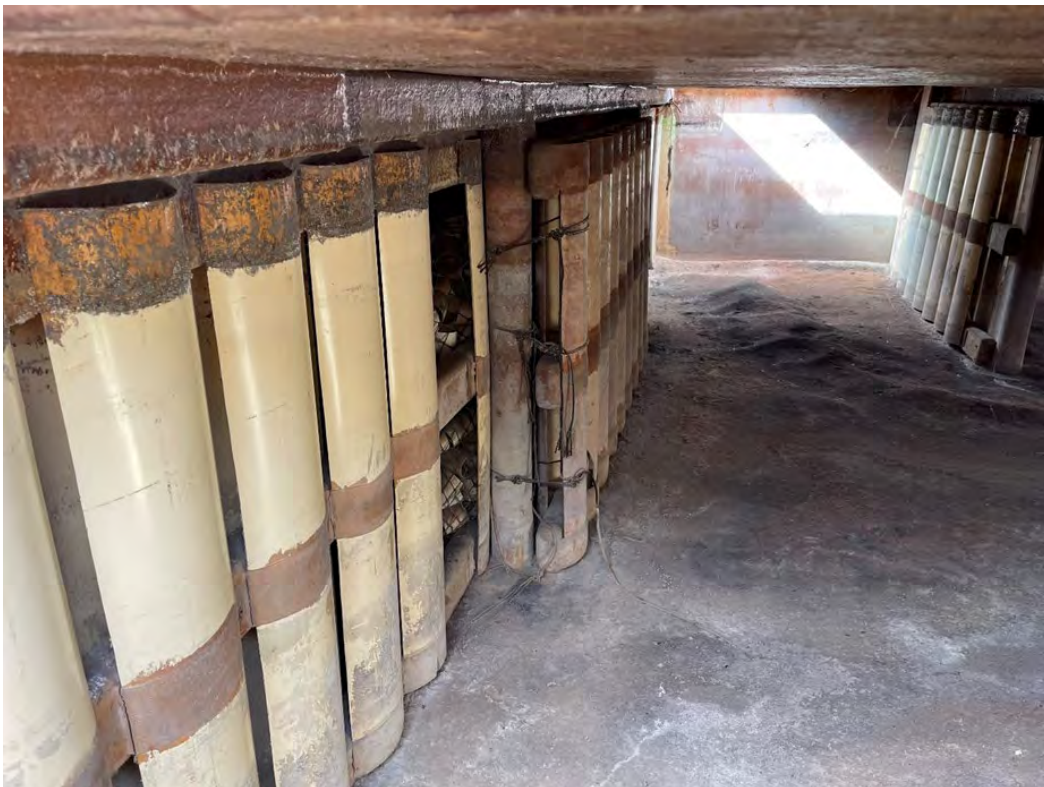
Image 1 / SX Mixer Settler cleanout lower level
