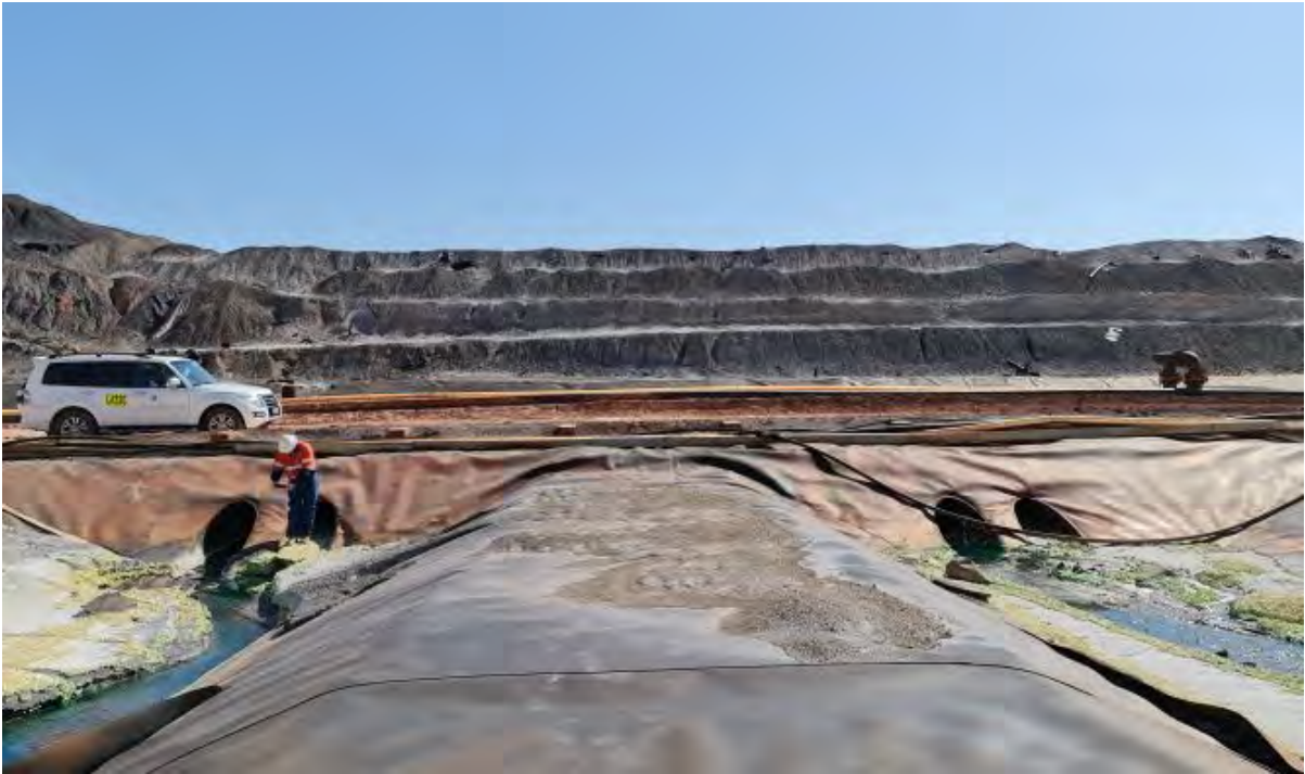
Image 9 / Leach Solution from Heap Drains – twin drains of copper sulphate solution
