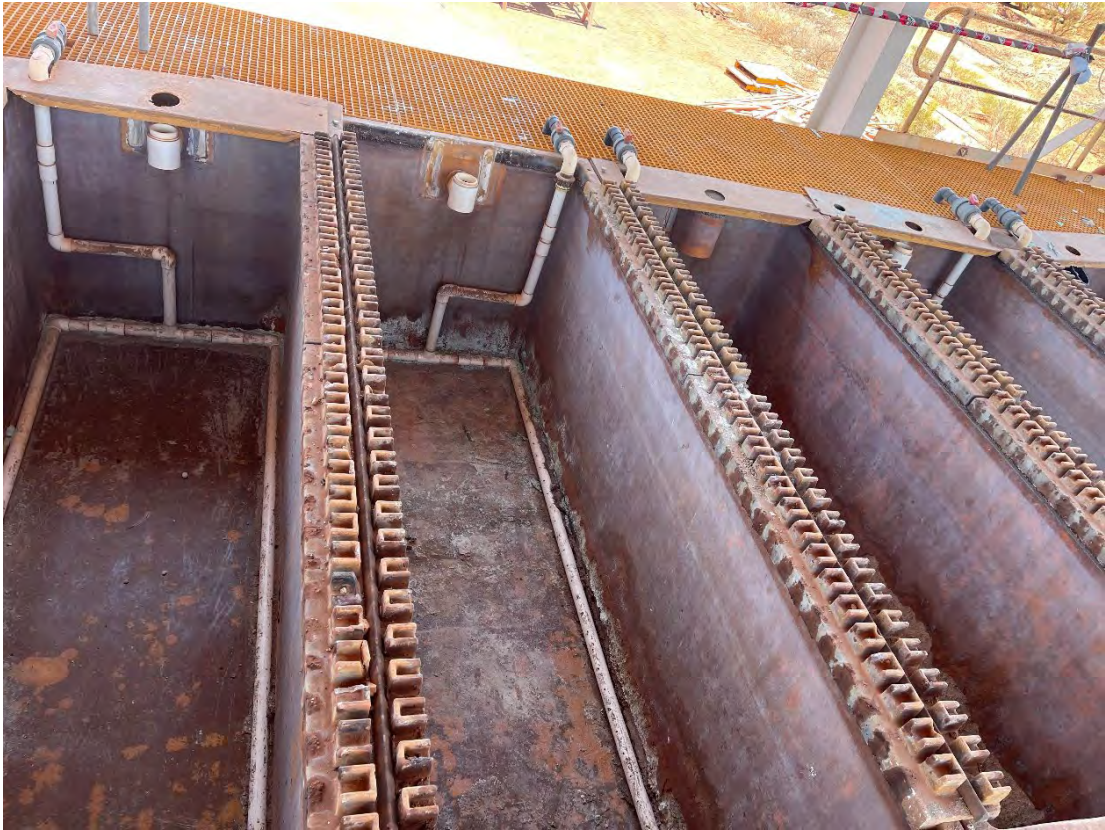
Image 4 / Cleaned EW Cells ready for condition inspection
