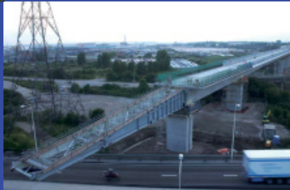
Right: Progress on the £178m Channel Tunnel Rail Link Contract 310 continued and in July 2003 Morgan-Vinci undertook one of the most complex launch stages of the 1km long Thurrock Viaduct, pushing the concrete deck in 45m long sections over the exit road from the Dartford Tunnel and beneath the QEII bridge at Thurrock.
