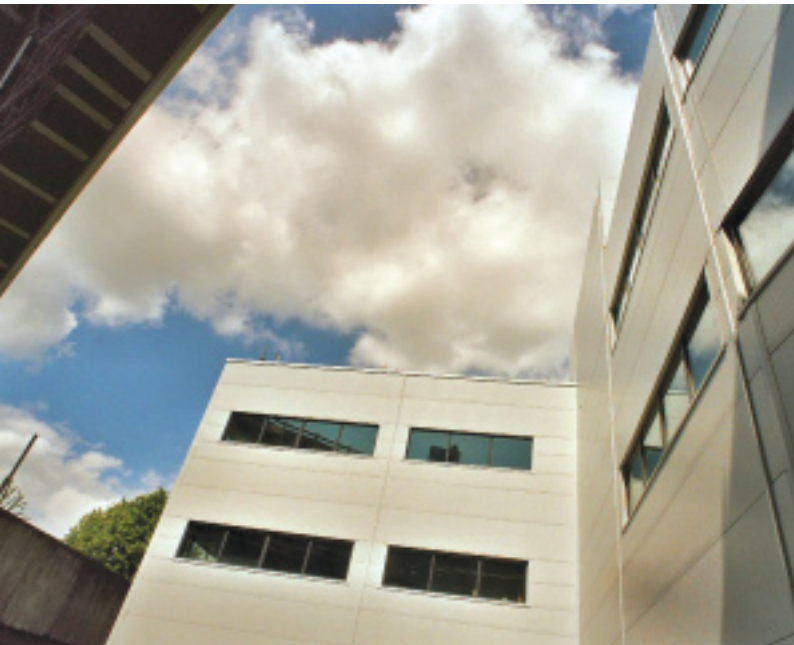
Left: The nation's first private walk in casualty centre built by Bluestone and fitted out by Morgan Lovell for private sector healthcare provider Casualty Plus opened in Brentford, West London. The three storey £5m centre allows patients with minor injuries to be treated immediately and avoid long waiting times in hospital accident and emergency.
