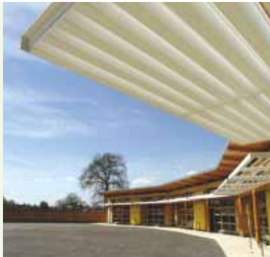
Above: Manor Green College in Ifield, Crawley, is one of two purpose designed special schools delivered by Bluestone in 2004 for West Sussex County Council within a £9m construction programme part funded by the Government's New Deal for Schools programme.
