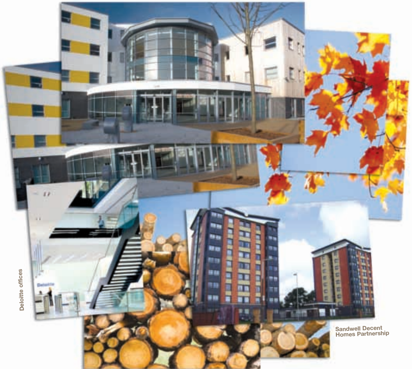
Radcliffe Primary Care Centre
