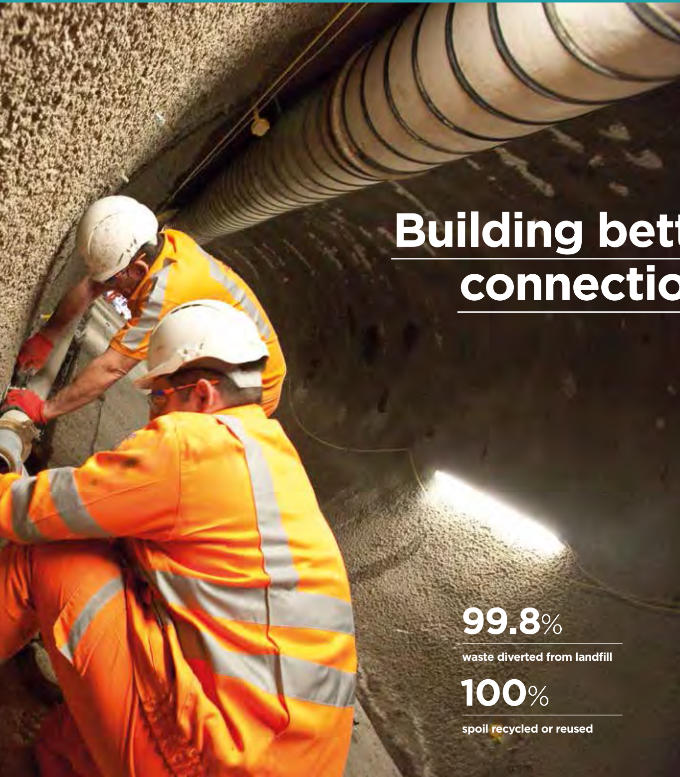
ABOVE: A sprayed concrete tunnel in progress on the C510 tunnels contract.
