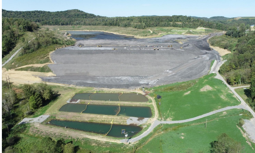
Figure 17-2: Coarse Refuse Stacker and Stockpile Area at Leer South (Photograph provided by Arch)
