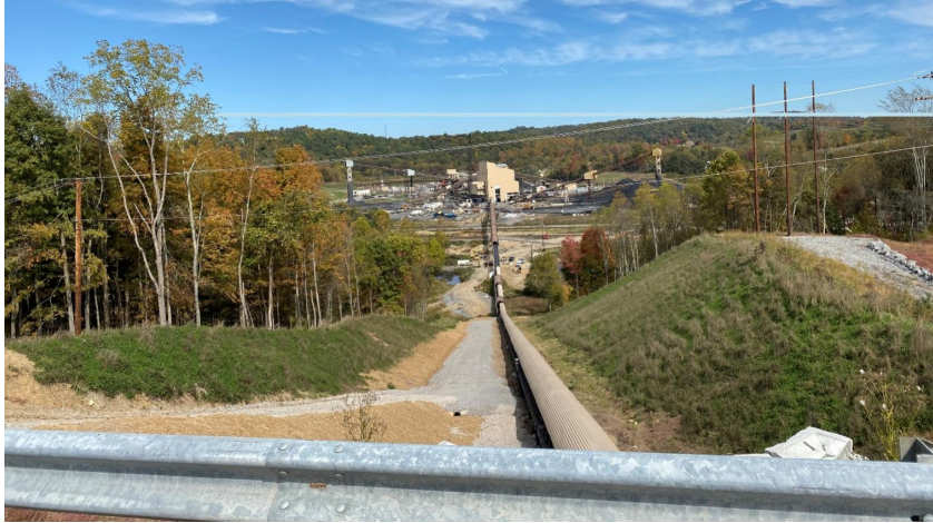
Figure 14-1: Leer South Preparation Plant as Viewed from Coarse Refuse Conveyor
