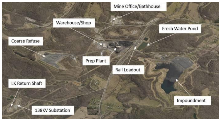
Figure 15-1: Leer South Surface Facilities
