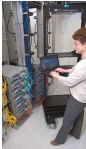
Test in progress using Avalanche NEXT.
