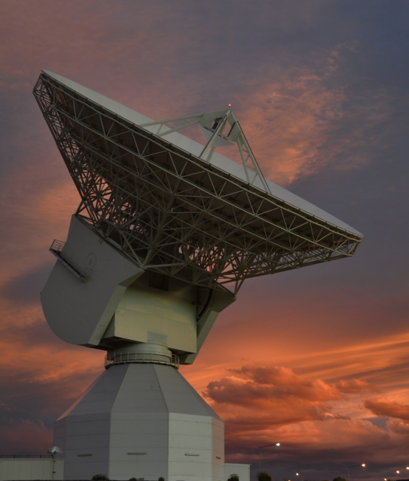
Systems Engineering provided the New Norcia antenna system, based in Western Australia, for the European Space Agency.
