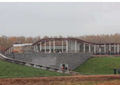
The Skolkovo substation
