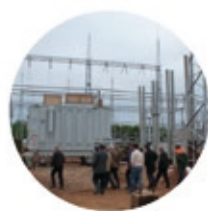
The ESPO Pipeline
