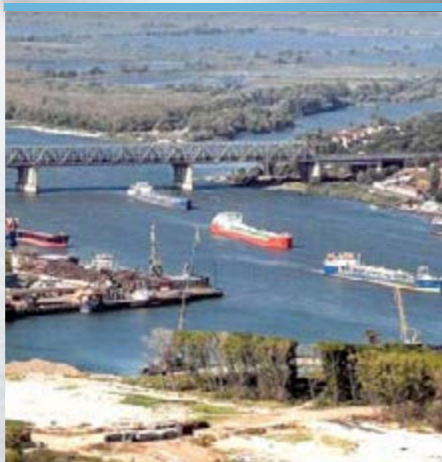
We reconstructed 220 kV Koysug SS (to 250 MVA), which will subsequently enable to provide reliable power supply to a number of large industrial consumer in Rostov oblast, such as JSC Rostovskiy Port
