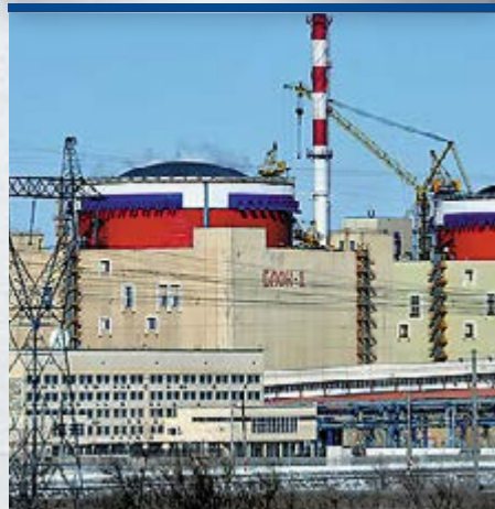
We commissioned 341.8 km of the 500 kV Rostov NPP – Tikhoretsk OHL, which is strategically important for the development of the South Federal District
