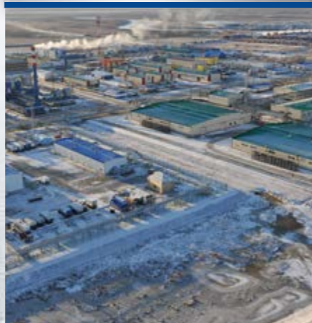
Our Company put into operation the second circuit of high voltage line between Urengoy HPP and oil fields of the Autonomous District with the total length of 426.7 km
