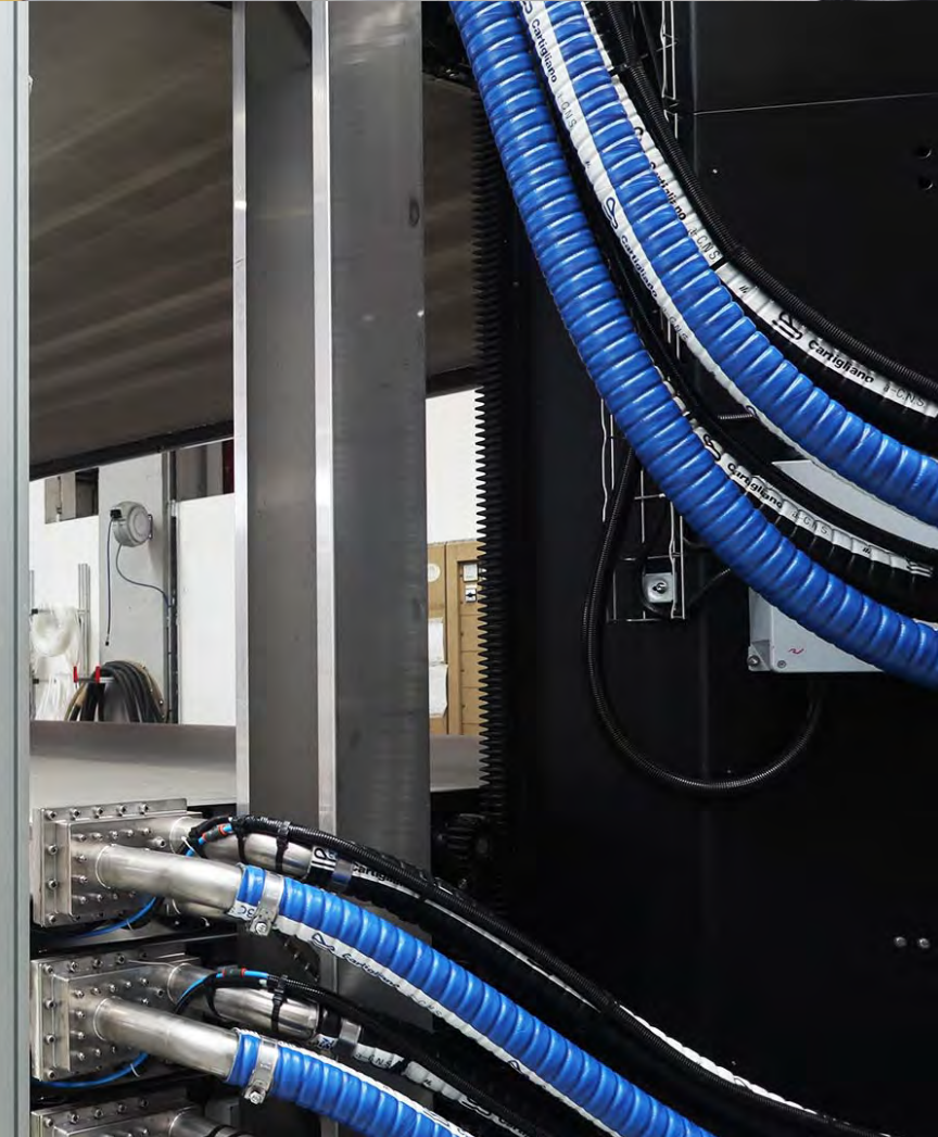
We continue to invest in capital equipment where an improvement in production efficiency, energy and water is apparent. In 2020, we initiated the purchase of: a new vacuum drier, three dye drum vessels, a whole hide splitting machine and two shaving machines.
