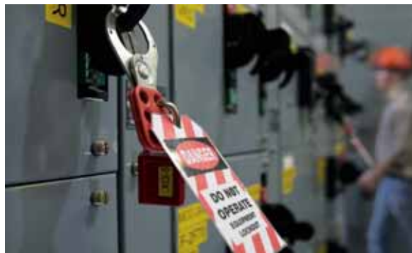
Our lockout-tagout system helps ensure the safety of everyone working on a piece of equipment.
