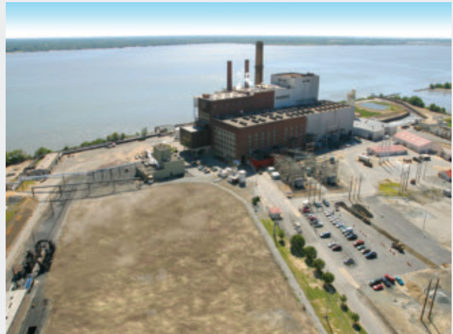
Edge Moor Energy Center (after)
