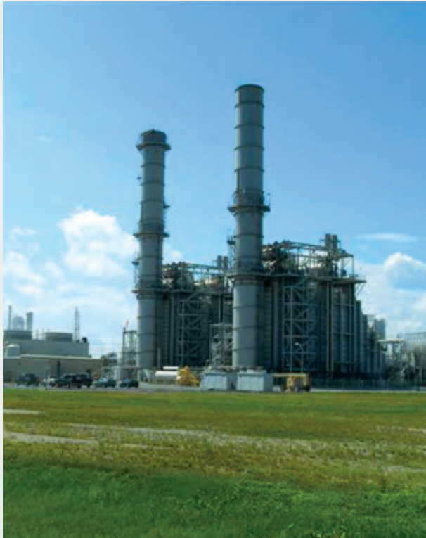
Carville Energy Center
