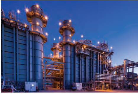
In 2013, we brought online more than 900 MW of combined-cycle capacity in California now operating under 10-year contracts, including our Los Esteros Critical Energy Facility.
