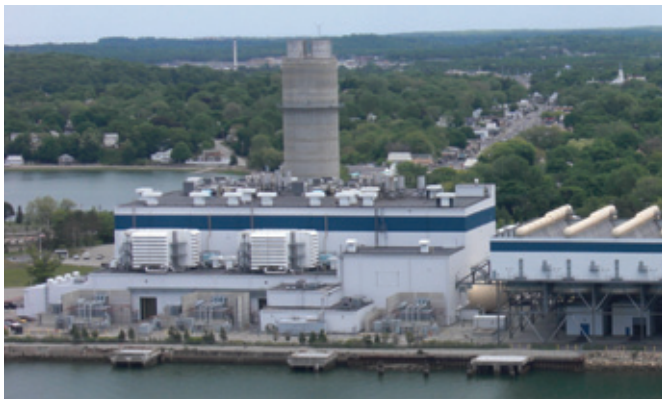
Our acquisition of the Fore River Energy Center in North Weymouth, Mass., expanded our footprint in the constrained New England market.
