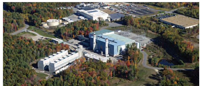
The addition of Granite Ridge Energy Center, an efficient, combined-cycle power plant in Londonderry, New Hampshire, has strategically increased our presence in the New England market.
