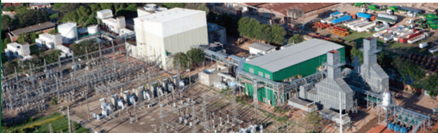
Photograph: Guaracachi Power Plant, Bolivia.
