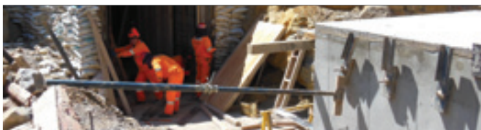
Photograph: Construction of tunnel three and collection chamber. Canchayllo, Peru.
