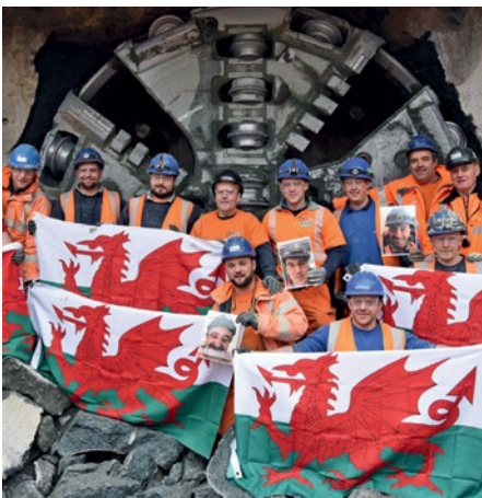
Break-through of the Bleddfa tunnel as part of the Birmingham Resilience Project
