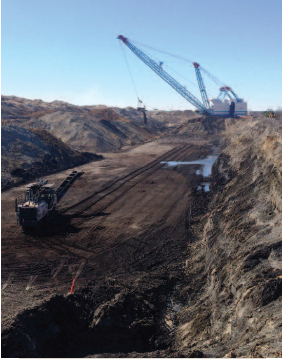
A new dragline and surface miner were put into service in 2014 at North American Coal's newest mine, Caddo Creek Resources Company, which commenced delivering coal in late 2014.
