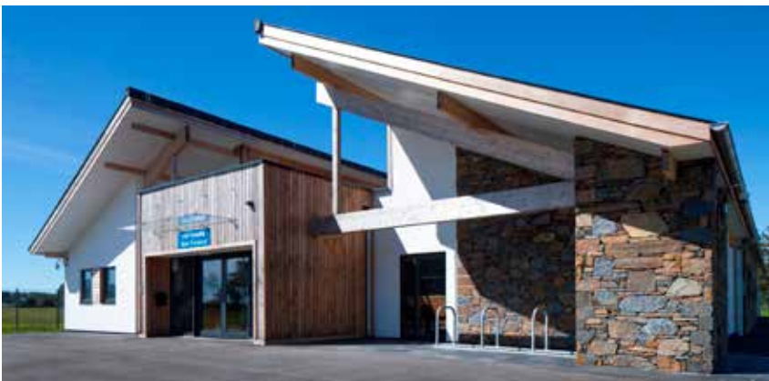
Arduwy Health Centre, Harlech Assura’s most sustainable property to date with an EPC rating of A+
