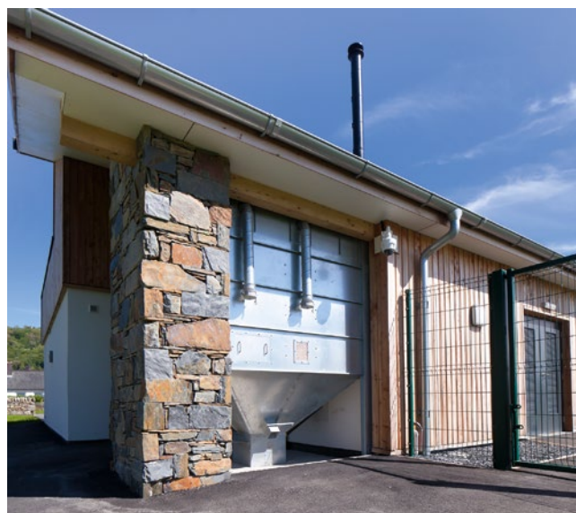
Arduwy Health Centre, Harlech
