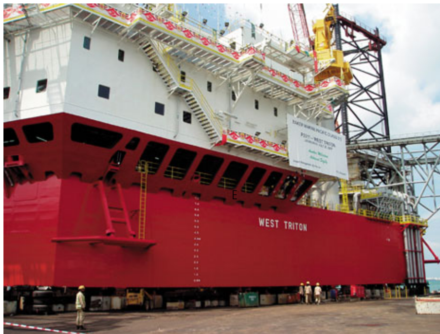
The West Triton Jack-up drilling rig under construction in Singapore
