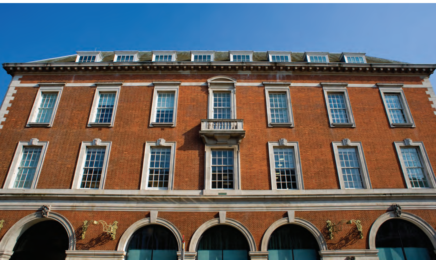
This page: 30 Kensington Church Street, London W8.
