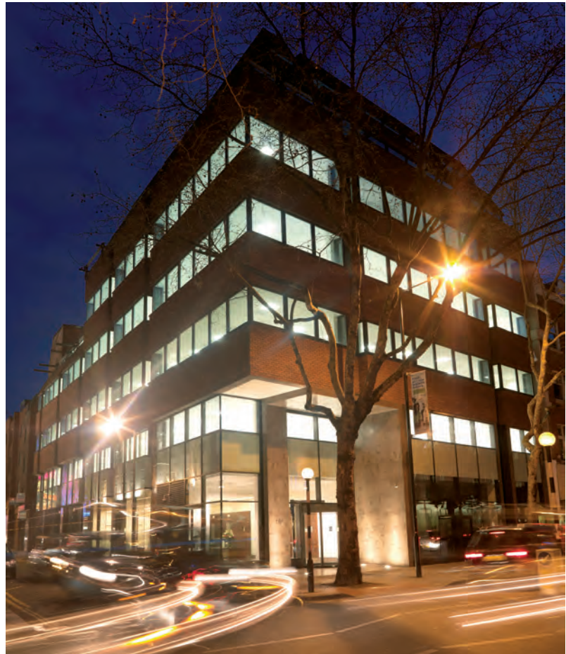
Right: 164 Shaftesbury Avenue, London WC2.
