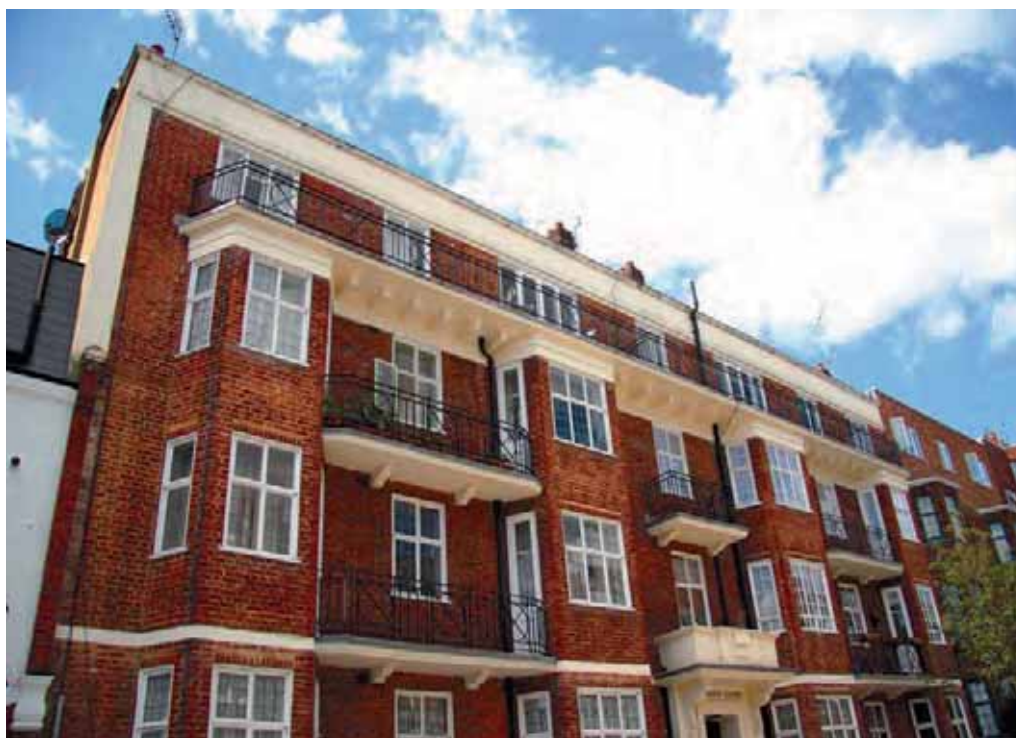
Above and left: Glenloch Court, London NW3. Opposite page: Oslo Court, London NW8.
