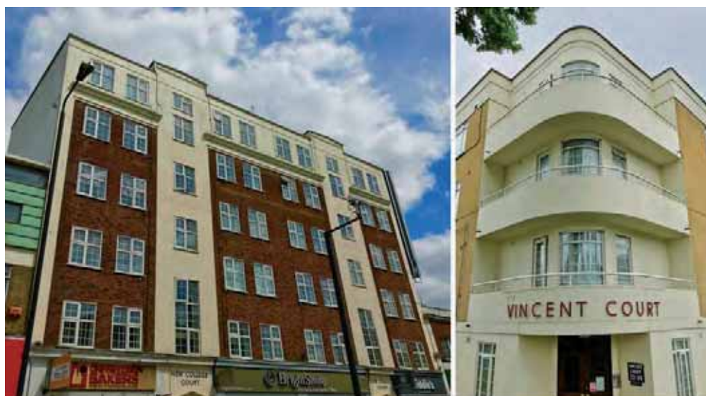
Above and opposite page: Grove Hall Court, London NW8. Right: New College Court, London NW3. Far Right: Vincent Court, London NW4.
