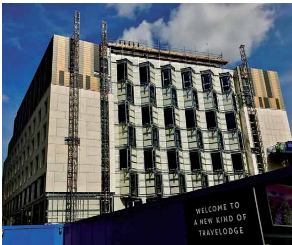
Right: progress on the Travelodge Hotel, Aldgate, London E1.
