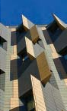
Above and background: the newly completed Travelodge, Middlesex Street, Aldgate, London E1.
