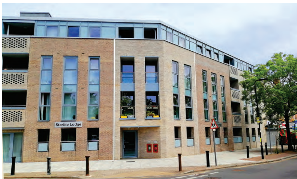
This page and opposite page: the recently completed Starlite Lodge, Greenford, Middlesex.
