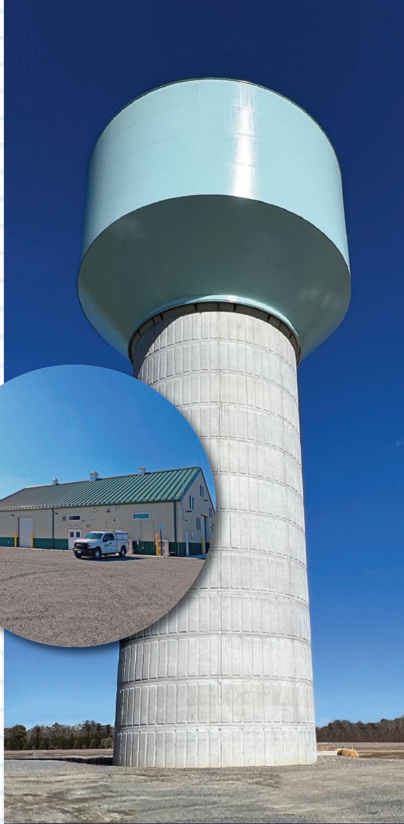
The Armory Road Water Treatment Plant and Elevated Tank provides an additional 1 million gallons of supply and storage to the rapidly developing southern Sussex County beach communities in Delaware.
