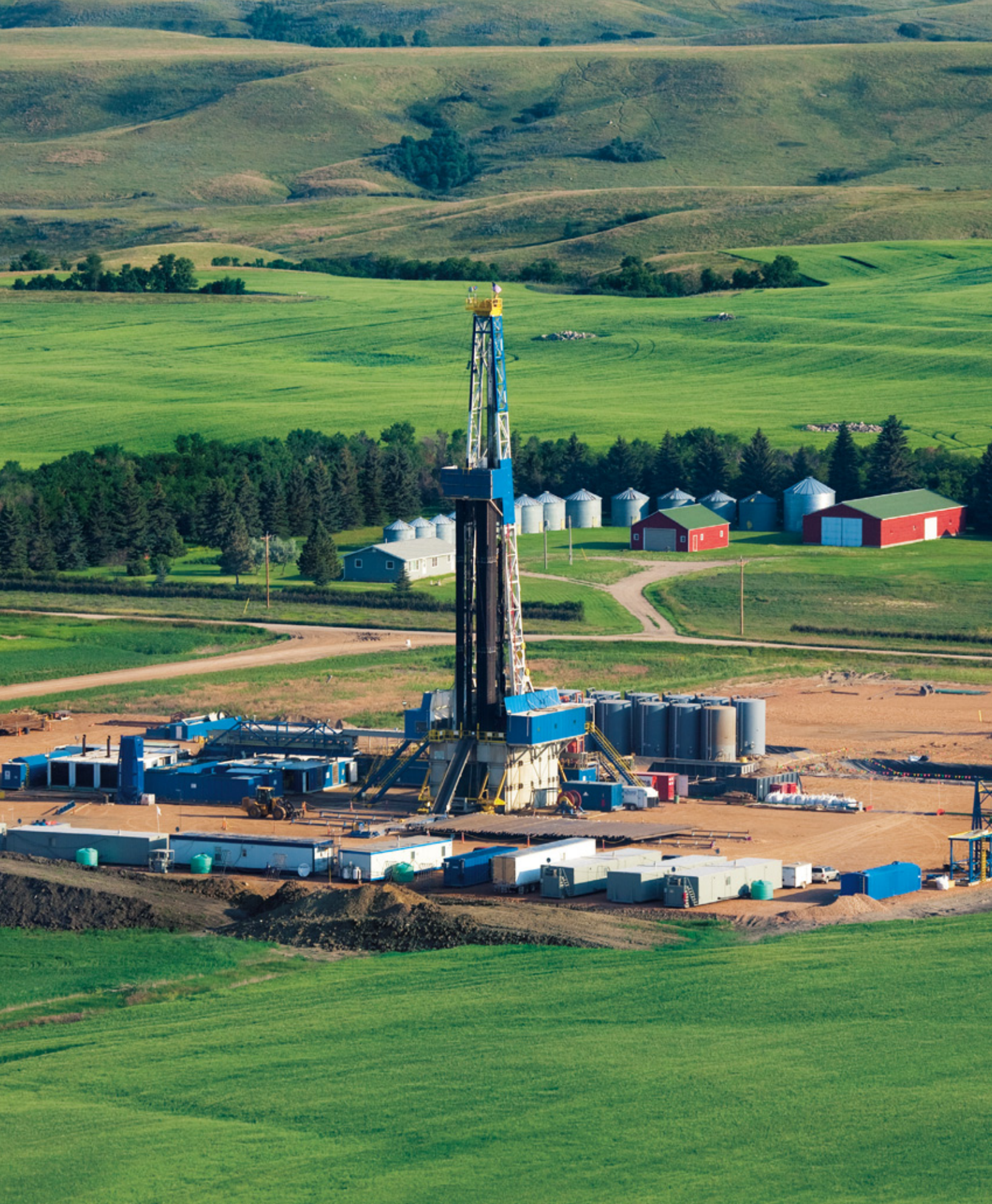
Drilling Operations, North Dakota
