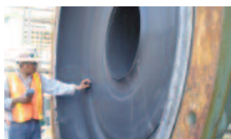
Checking the wear rate on the rubber liners in a Warman MCR Mill Circuit pump.
