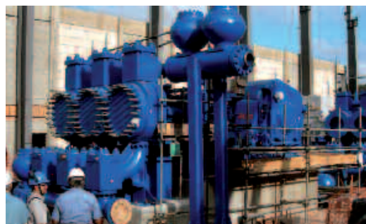
Geho pumps being installed on the Brazilian pipeline.
