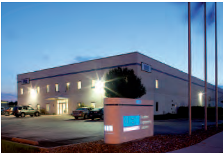
Weir Oil & Gas Services, Deer Park, Texas
