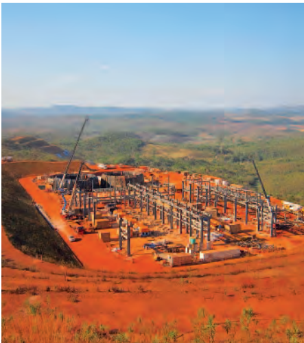
GEHO® pumps in place at the Anglo Ferrous iron ore mine in Brasil, the world's biggest pump station
