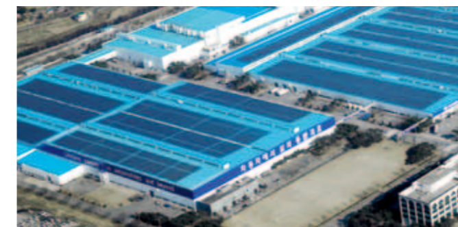
The Solar Power Plant at the Asan plant
