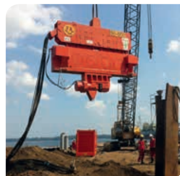
Onshore Vibratory Piling
