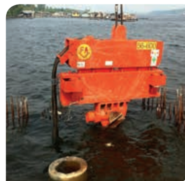
Offshore Vibratory Piling
