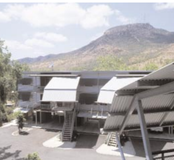
LEFT: BUILDINGS SUCH AS THE LAVARACK ARMY BARRACKS IN TOWNSVILLE HIGHLIGHT THE ENVIRONMENTAL CREDENTIALS OF STEEL
