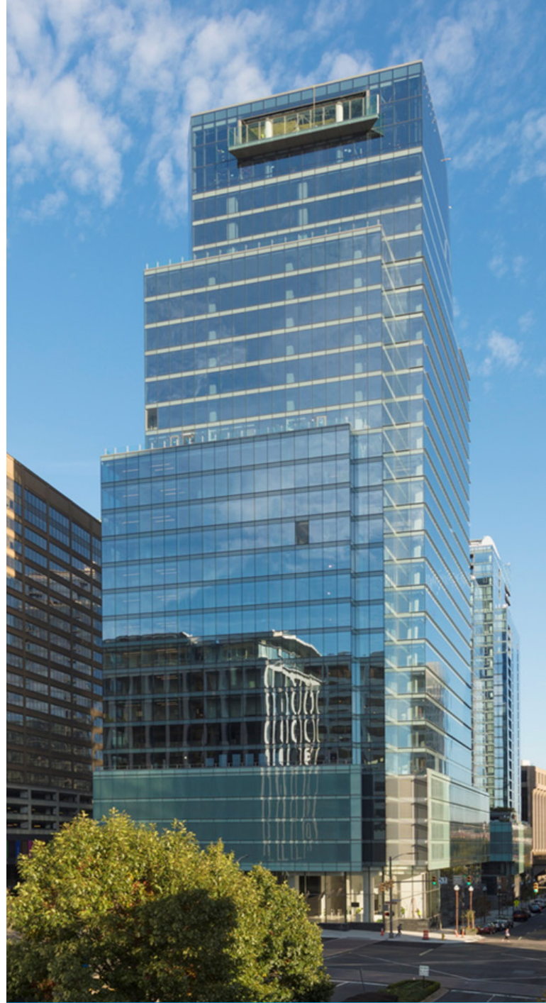
CEB Tower at Central Place
