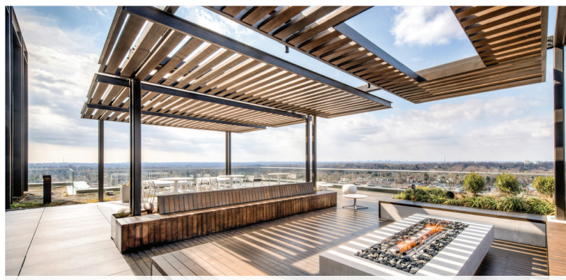
4747 Bethesda Avenue (Rooftop)
