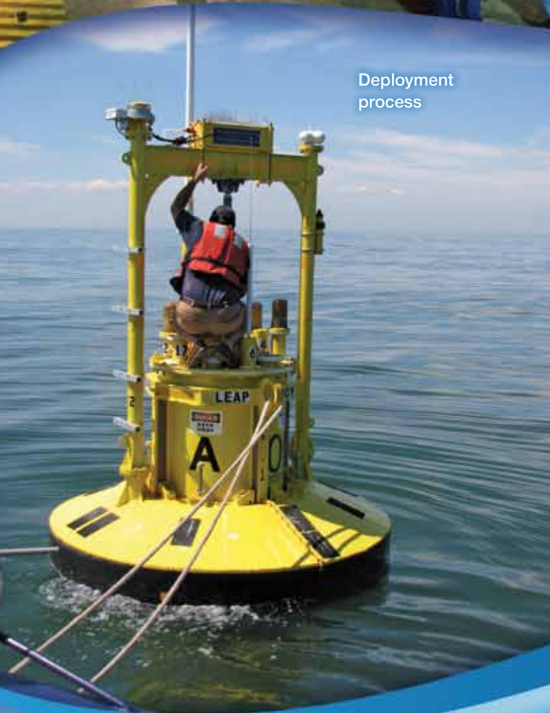
Final systems check
