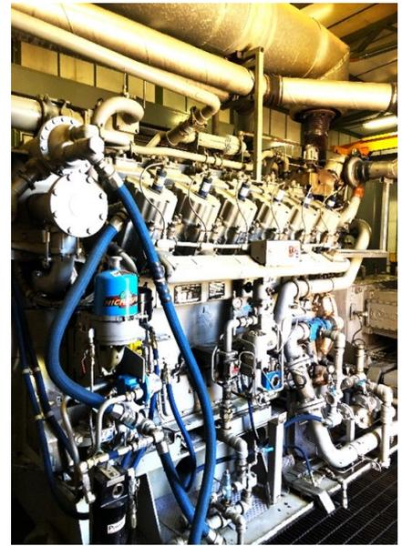
*Part of the newly acquired RPGP – low pressure gas is compressed to sales gas pressure using gas engine driven reciprocating compressors*
