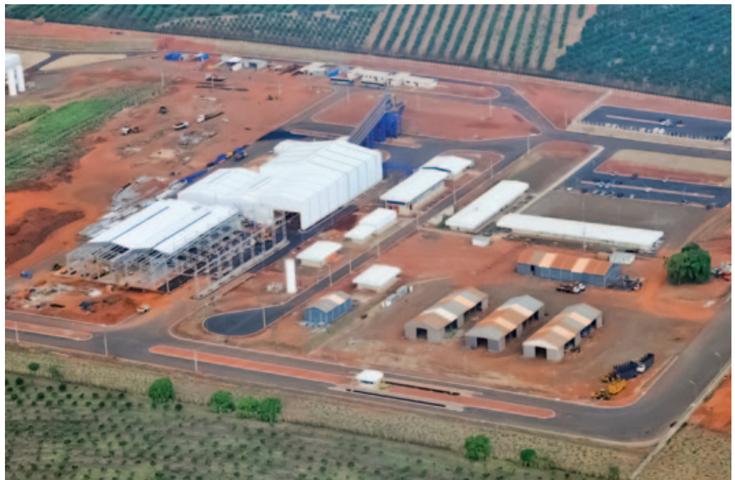
Purpose-built facility for PLENE ® production in Itápolis, Brazil.
