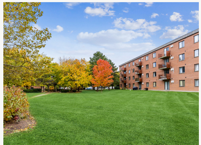
Northfield Gardens WATERLOO
